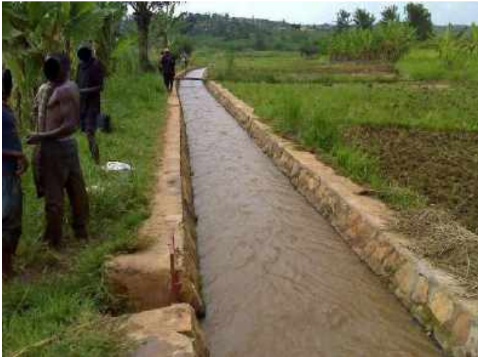
Figure 19: Functional irrigation canal in the province of Cibitoke.
